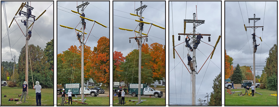
Contractors specializing in transmission line work are seen here reconfiguring a transmission structure on the 69 kV transmission line in October 2016. Such reconfigurations were done with the line energized, to minimize the number and length of planned transmission-line power outages.
