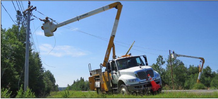
EMEC linemen running wire to a new line extension across Route 1 in Perry.
