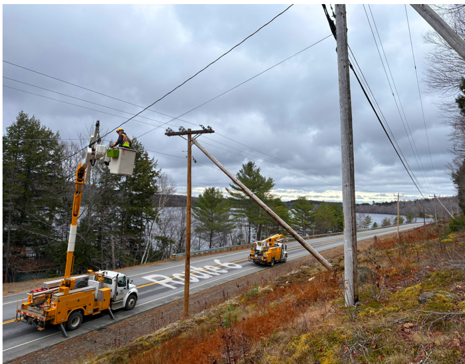
This stretch of the Springfield circuit along Route 6 was originally constructed on the side of a hill. By moving the line closer to the road, EMEC crews have made faster repairs possible. This will also lower the cost of maintaining and upgrading the line.
