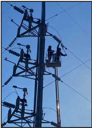
EMEC linemen replacing a high-voltage insulator during a planned outage at the Woodland Substation.
